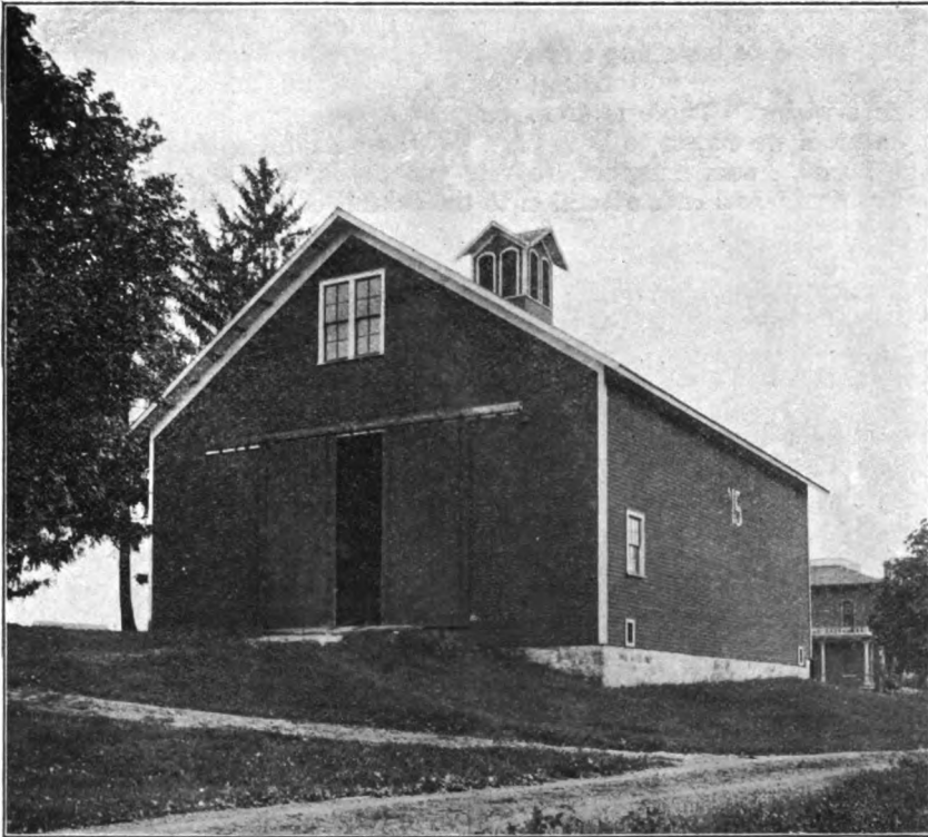
Barn for the Experiment Station.
